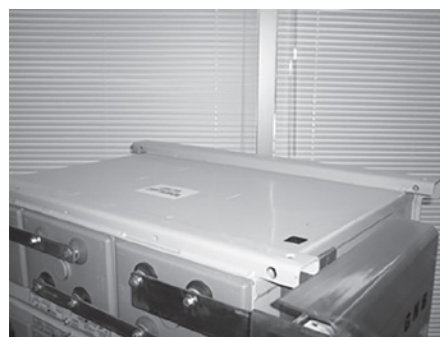
Figure 4: Recommended Frame Ground Location
