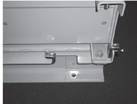
Figure 1: Beam Clamp Installation
