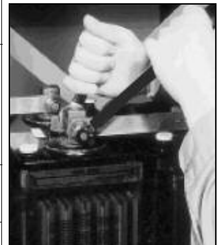
FIGURE 1.4.7 - Torquing connections
