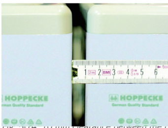
Fig. 5-14: 10 mm clearance between the batteries
